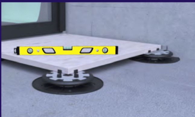
4. Slab levelling
